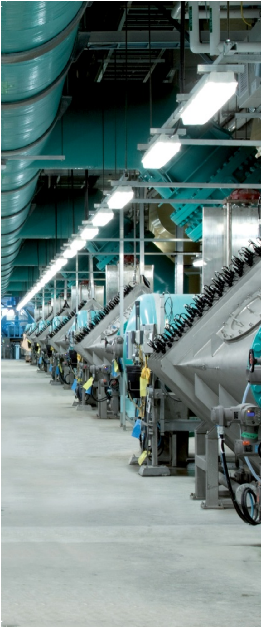
24 WEDECO K 143 UV disinfection systems at Vancouver's Seymour-Capilano Filtration Plant treat up to 1.8 billion liters per day, making it one of the largest UV disinfection facility for drinking water in the world
